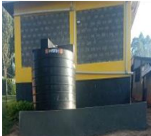
.....the tank installed
