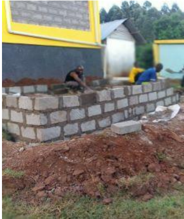
The foundation base built
